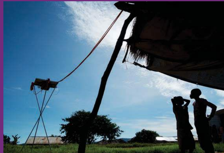
PHOTO: Wires connecting Devergy households / CREDIT: Devergy
