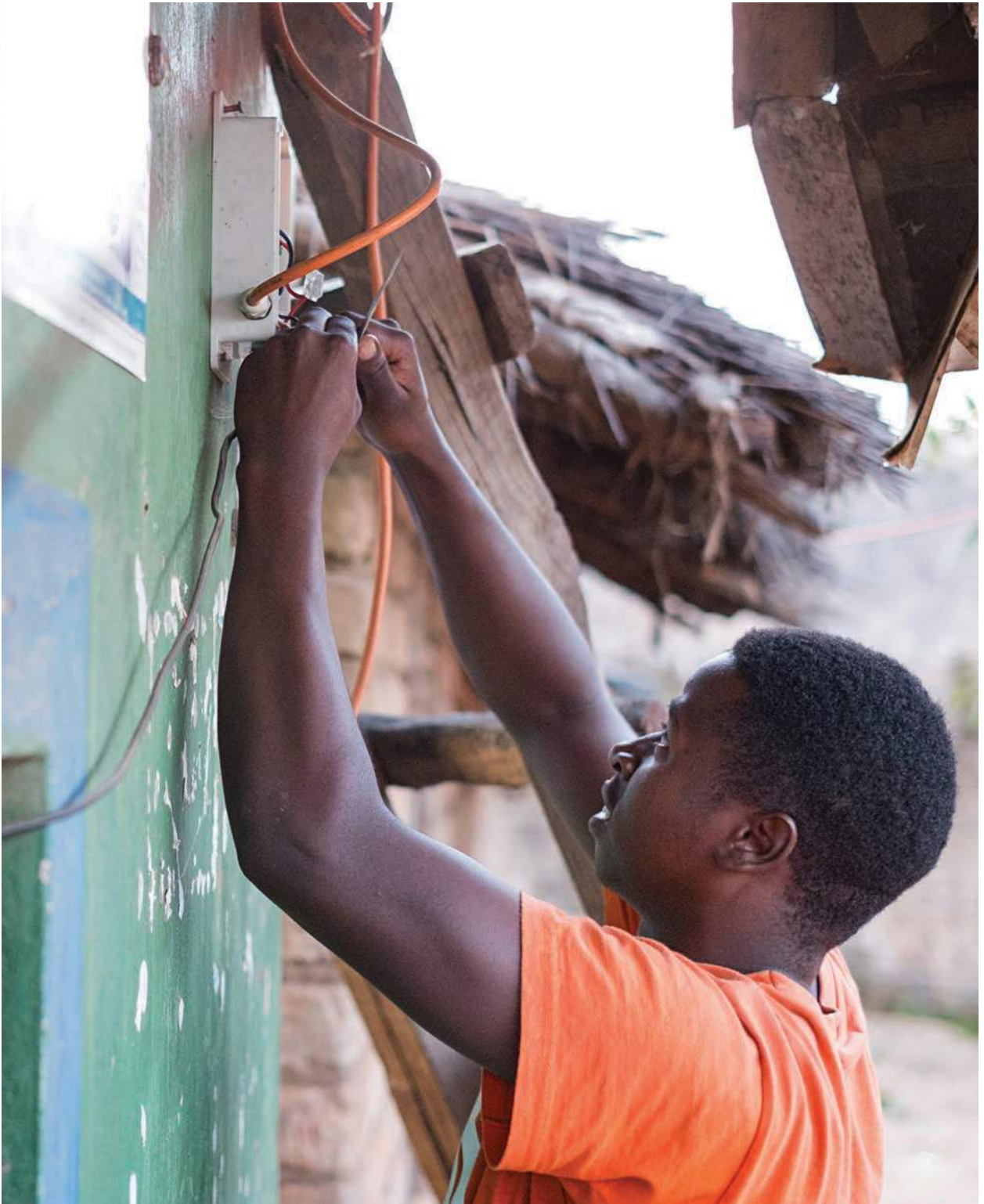
PHOTO: Installing a meter for Devergy / CREDIT: Devergy
