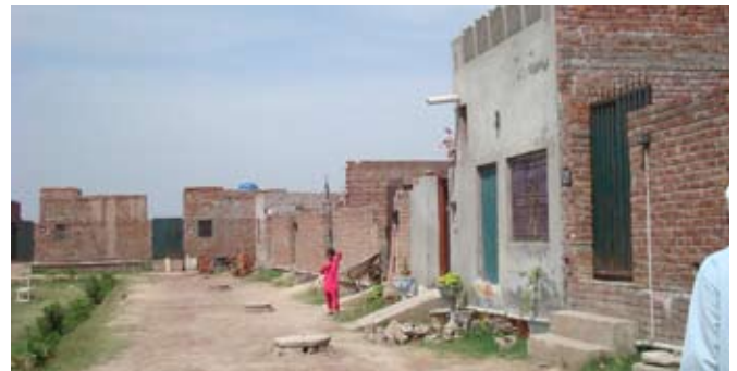
A row of homes in Block A of KKB-4
